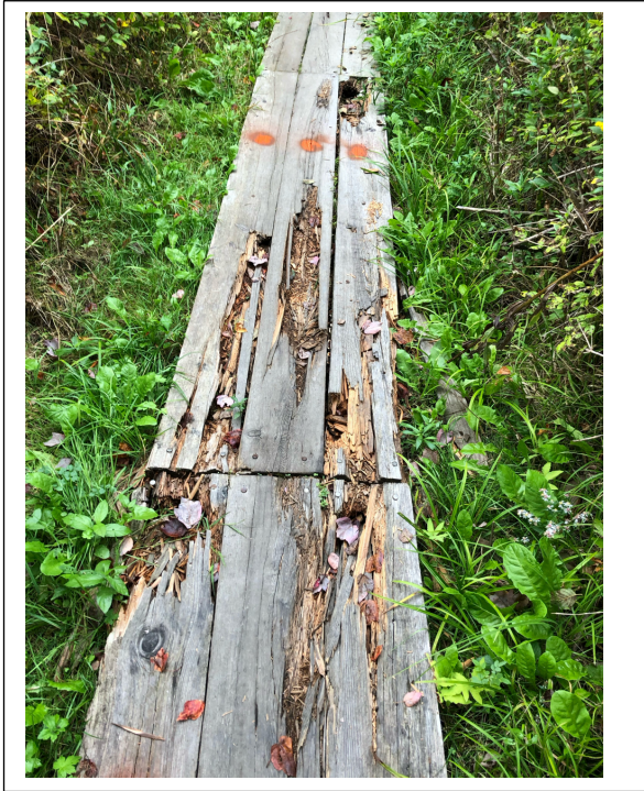
Boards on the Outer Loop Trail marked with orange paint and ready for replacement boards.
